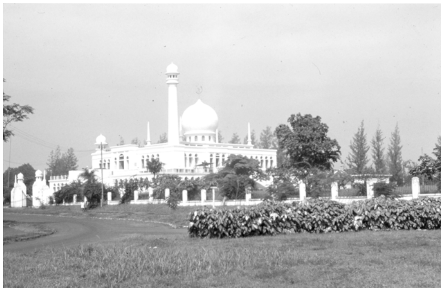
Al-Azhar mosque, Kembangan Baru, Jakarta, built after independence and reflecting Middle Eastern influences.
