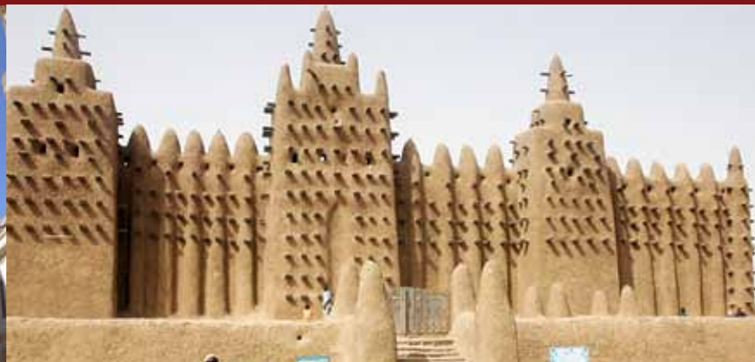
Djenné is home to the world's largest mud mosque. This is more impressive than it may sound: the building is huge, and manages to be elegant both up close and from a distance. Two times a year all the city's residents drop everything, cart mud up from the nearby Bani river, and together they re-pack the Mosque walls.
